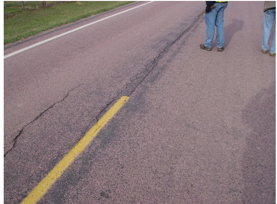
Longitudinal and centerline cracking
