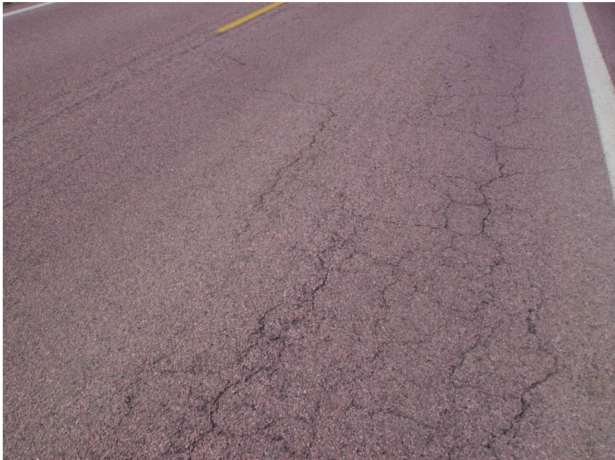
Fatigue Cracking Section SS2
